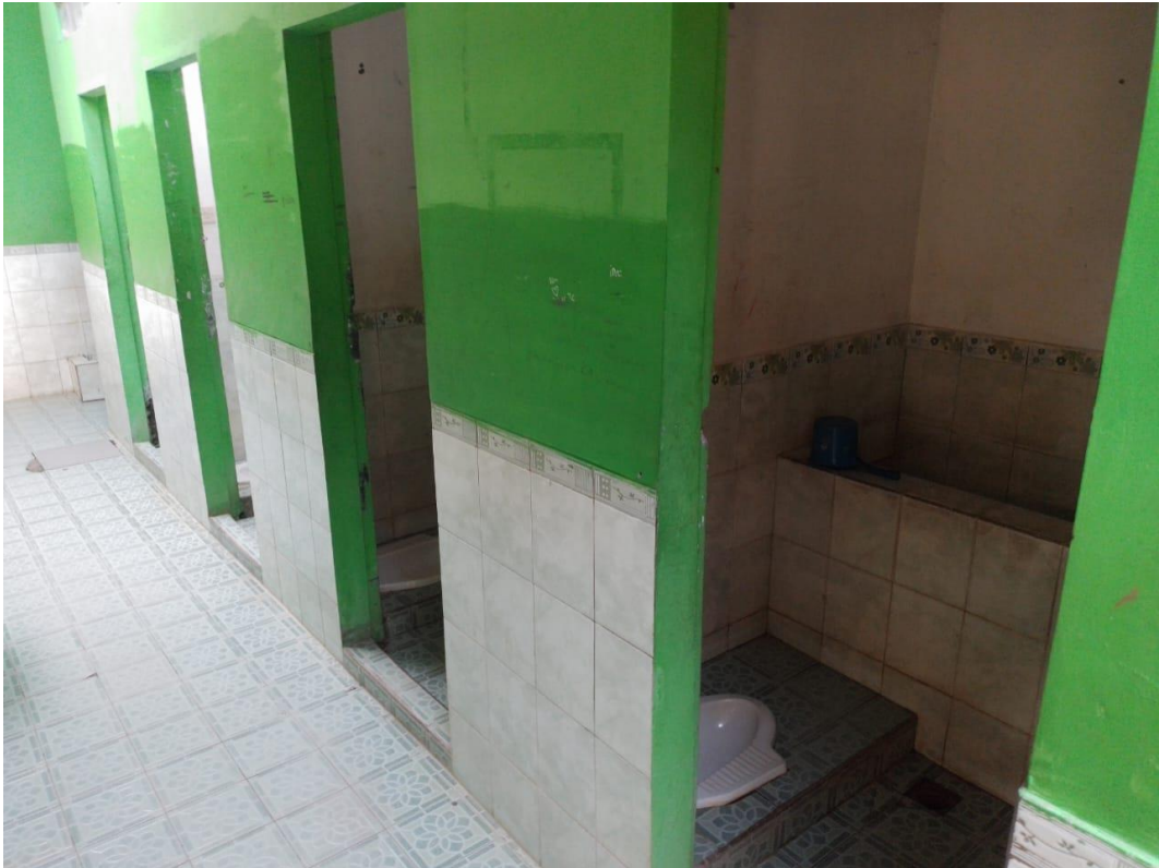
Kamar Mandi MTs Raudlatul Huda Adipala
